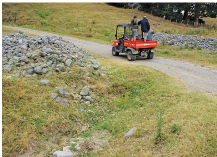
The brothers also upgraded culverts to prepare for future storm events.
